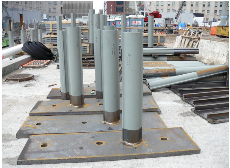
Figure 37: Security bollards are to be embedded around the WTC site to prevent vehicles from entering (own photography Fraunhofer EMI)
