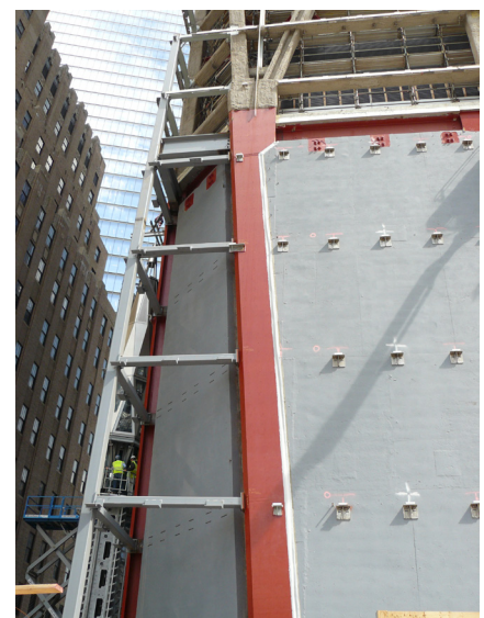
Figure 36: Reinforced building pedestal of One World Trade Center (own photography by Fraunhofer EMI)
