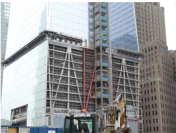
Figure 36: Reinforced building pedestal of One World Trade Center (own photography by Fraunhofer EMI)
