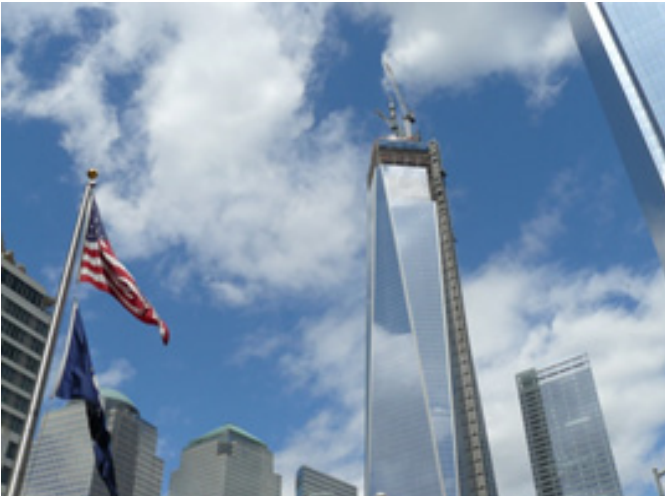
Figure 33: View of One World Trade Center tower (April 19, 2013); construction elevator attached onto tower (right) (own photography Fraunhofer EMI)
