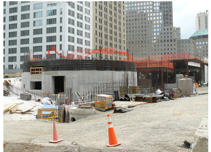
Figure 35: Entrance to the VSC; helix pathway directing vehicles to the parking zones (own photography by Fraunhofer EMI)
