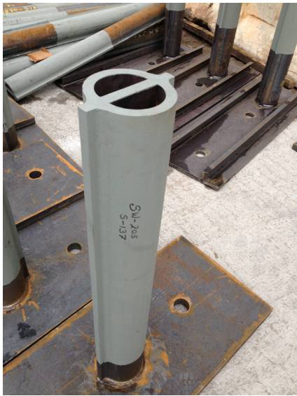
Figure 37: Security bollards are to be embedded around the WTC site to prevent vehicles from entering (own photography Fraunhofer EMI)
