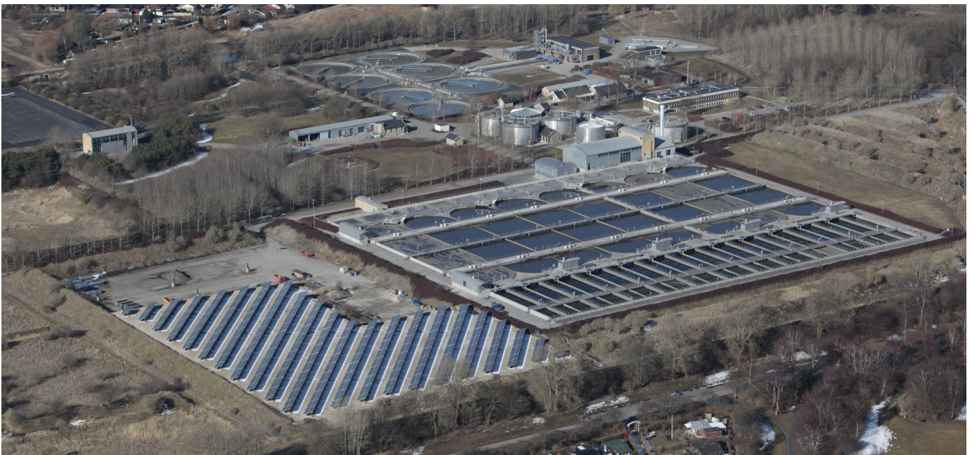
Figure 38: Large scale PV plant on top of the waste water sludge deposit (© Jakob Klint, Kuben Management A/S 2013).
